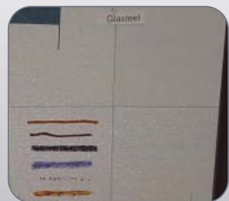
After Stain Cleaning Test
